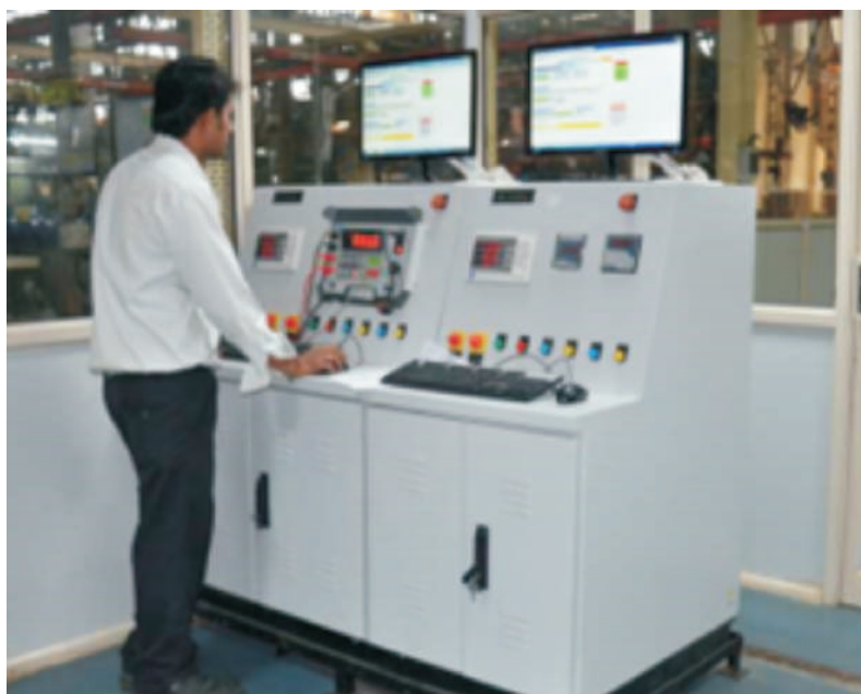
SCADA Test Facility
